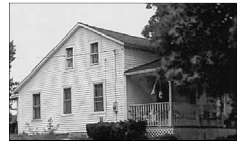
Top photo: Home of John Y. Johnson in Johnnycake Hollow destroyed by fire in 1854 Bottom photo: Home rebuilt after fire present home of Dan and Kari Houchen
